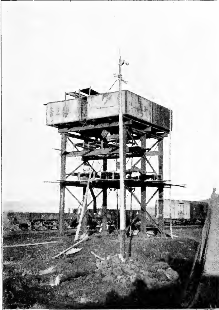
“PERCHED ON THE TOP OF WATER-TANKS.”
